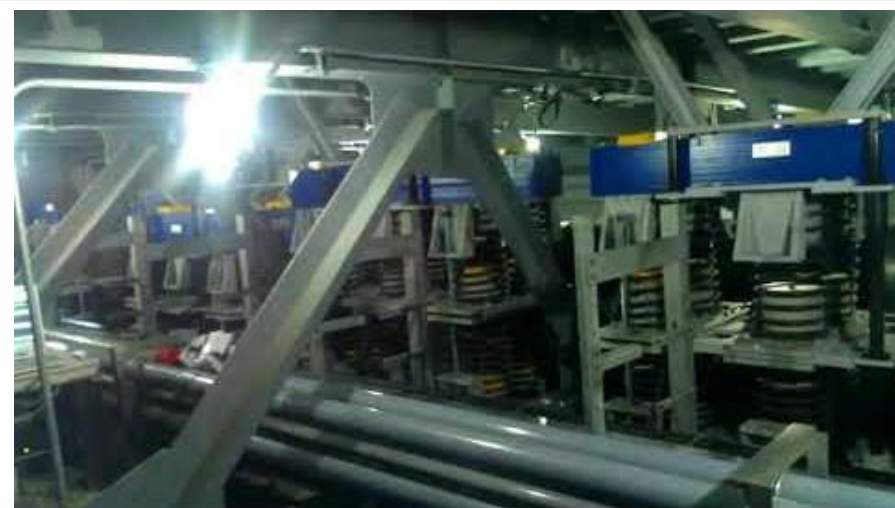
FIGURE 4.4: Tuned mass damper with spring and damper assemblage.
